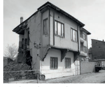
The front facade of Konya house in Mahmutdede Avenue (First half of the 20th century).
